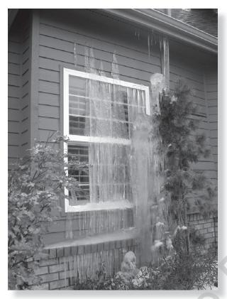
**Figure 1-13** A broken pipe on a second floor caused a massive water leak in this home. The water eventually made its way into the exterior walls and behind the siding, resulting in this rather dramatic ice sculpture in the front yard.
