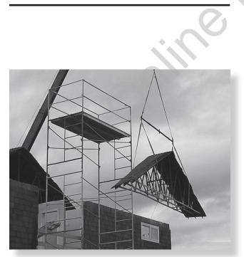
*Figure 1-11* Structural repairs, such as those for this firedamaged roof, can be quite involved. They make up the second part of insurance restoration work.
