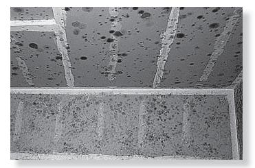
*Figure 1-15* Mold is a tough and often dangerous problem in water-damaged homes. Many insurance restoration contractors also offer mold remediation services.
