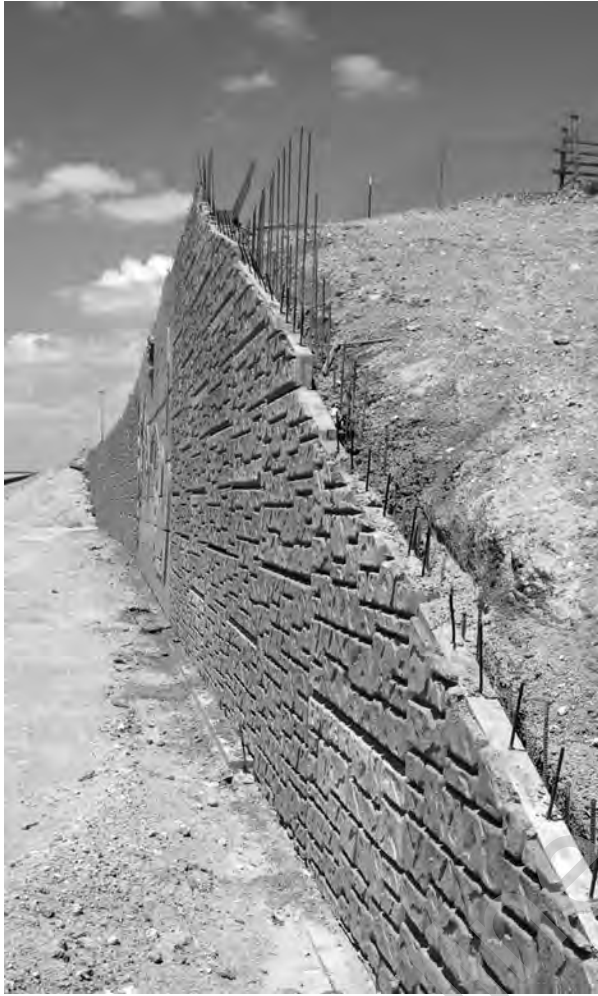
Figure 1-2 Concrete panels that replicate natural stone
