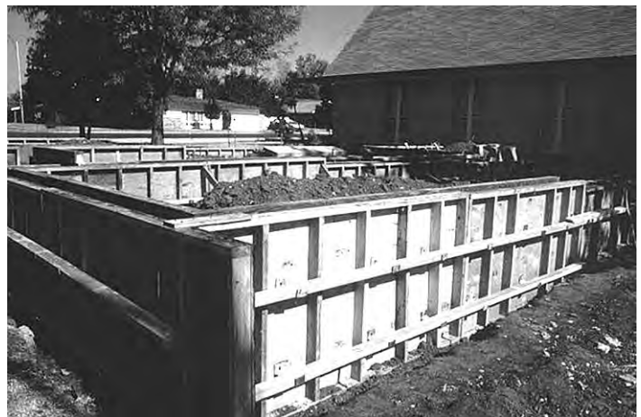
Figure 1-4 Poured concrete wall forms
