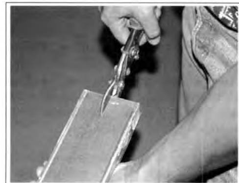
Figure 1-27. Cutting the slice in one end of a stick of 3 5 / 8 -inch plate, using snips.
