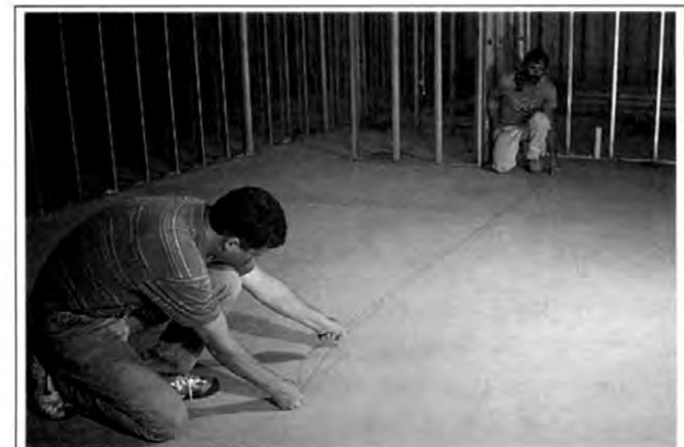
Figure 1-16. Here the chalk line has been set and is ready to snap.
