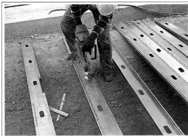
Figure 1-73. Cutting down the hard side of a structural stud using a Quickie Saw.
