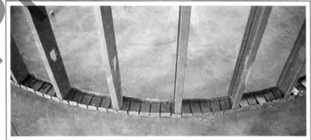
Figure 1-80. A standard 3\frac{5}{8} -inch plate with relief cuts made approximately every 2 inches is shot to the floor.
