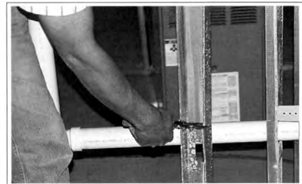
Figure 1-66. Marking the notch with your snips, as shown here, is much faster than measuring and marking the cut with your tape and marker.
