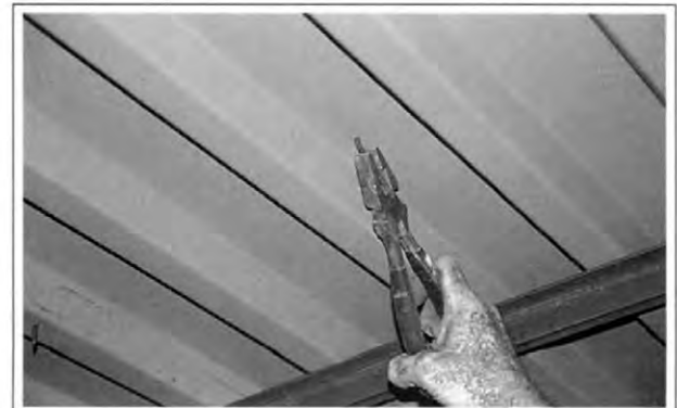
Figure 1-42. Grab a long decking screw near its base with lineman's pliers and bend it over, snapping it off.
