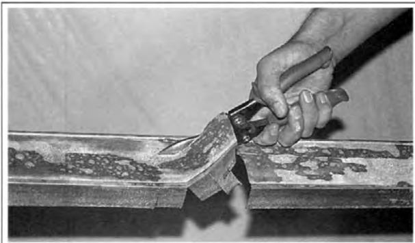
Figure 1-69. The relief cuts allow the scrap stud to roll up out of the way as the notch is cut out of the stud.
