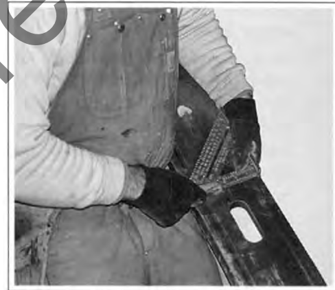
Figure 1-26. Using a speed square to "score" a 6-inch structural stud with a utility knife. The stud sometimes needs to be scored several times. The better it's scored, the quicker it will snap off when you fold it back and forth.
