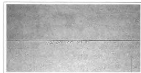
Figure 1–13. The rough opening for a window laid out along the wall line, telling the carpenter that the window R.O. is 42 inches off the finish floor and 40 x 40 inches.
