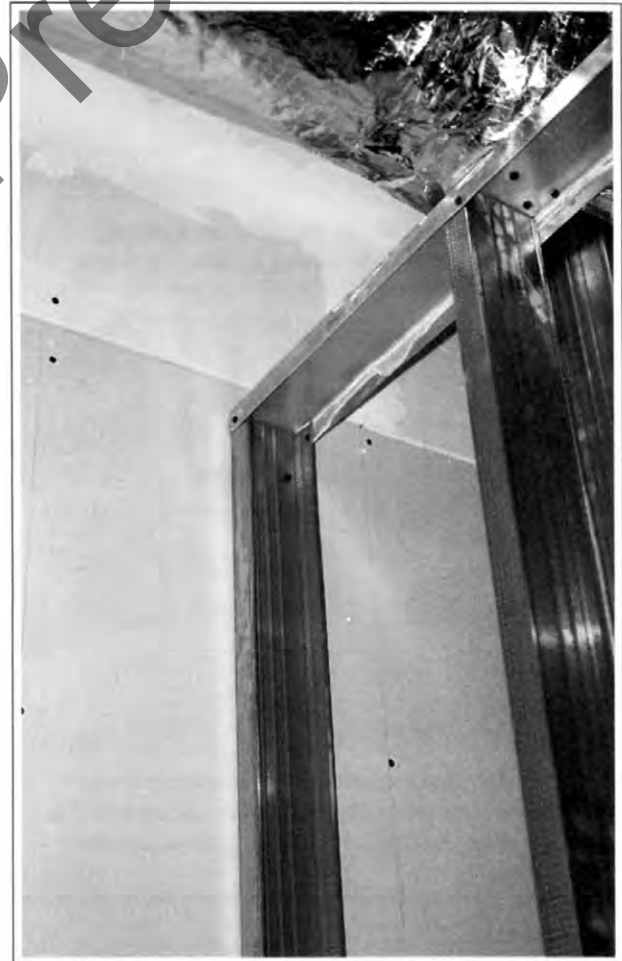
Figure 1-54. The first stud of this wall was tied into an already-framed and -rocked wall. Then the top plate of this wall was screwed off to the stud to start the wall. The first stud of a freestanding wall like this can also be shot to structural steel or block walls.
