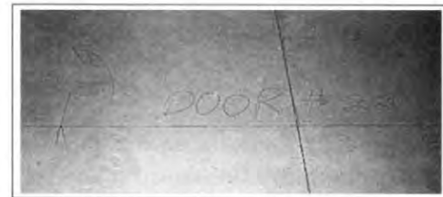
Figure 1–12. A door laid out along the wall line with the door number and swing marked out in the door opening.
