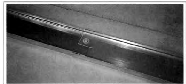
Figure 1-31. The ends of two sticks of bottom plate spliced together and shot down with one pin.
