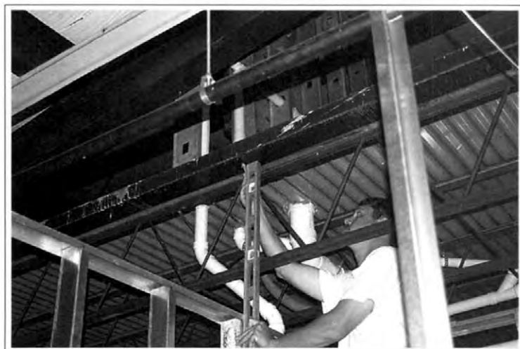
Figure 1-95. Using a level to transfer the wall line of a wall framed to the bar joist on up to the deck.
