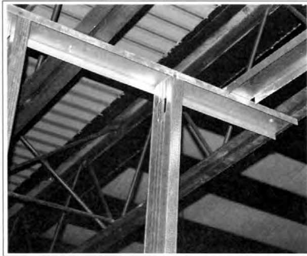
Figure 1-46. The top plate of a 3\frac{5}{8} -inch wall run past the actual corner point to the next bar joist and shot in place, with the top plate of the intersecting wall tabbed and set in place.
