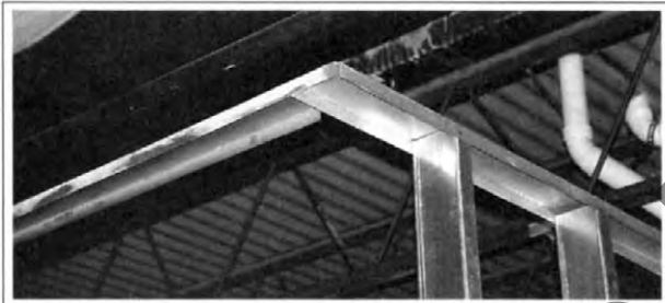
Figure 1-49. You can see the plate set in place overlapping the first stick of plate to form the corner.
