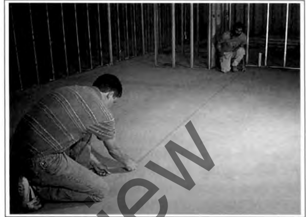
Figure 1-14. In this example you see the chalk line being pulled well past the far crow's-foot, and adjusted to the crow's-foot.
