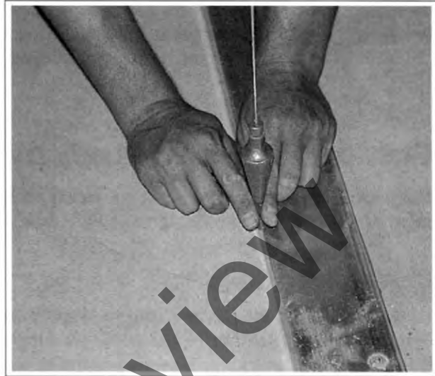
Figure 1-18. Steadying the tip of the plumb bob with light, even pressure from each index finger.
