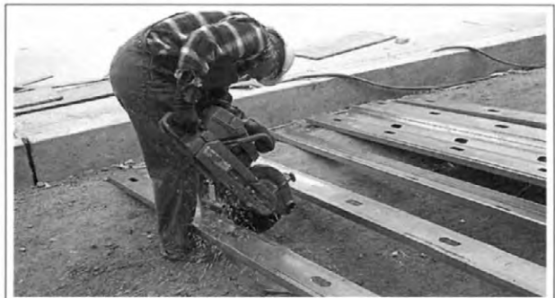
Figure 1-71. Using a Quickie Saw to make the first two cuts of the notch in a structural stud.
