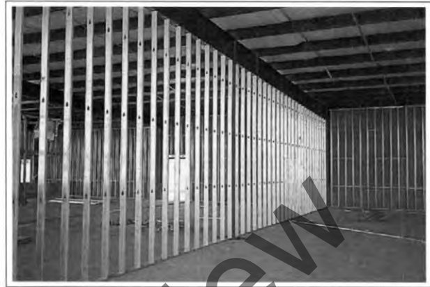
Figure 1-61. Here's a typical 3\frac{5}{8} -inch wall framed up, with all the stud holes lined up.
