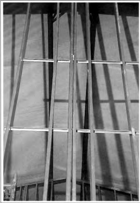
Figure 1-93. With the expansion studs stood up and the layout studs in place, pieces of CRC have been cut to span two layout studs on either side of the expansion. The CRC keeps the wall solid at the expansion.
