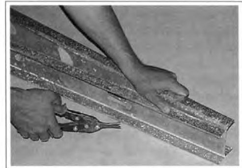
Figure 1-23. A stud cut square, using snips. You can tell if the cut is square by folding the stud back over and making sure the edges of the stud line up.
