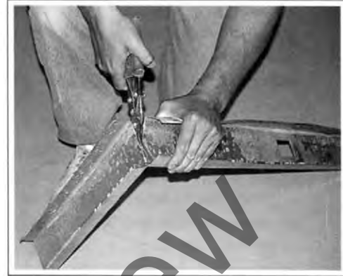
Figure 1-25. The scrap side of the stud rolls up out of the way if you grip it tightly, allowing the snips to easily pass through the cut.
