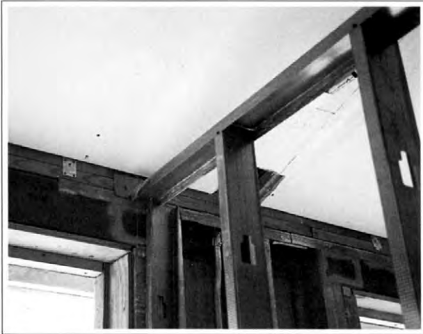
Figure 1-55. Here's the top plate of a freestanding wall fastened in place using a shoe turned up and flattened out.
