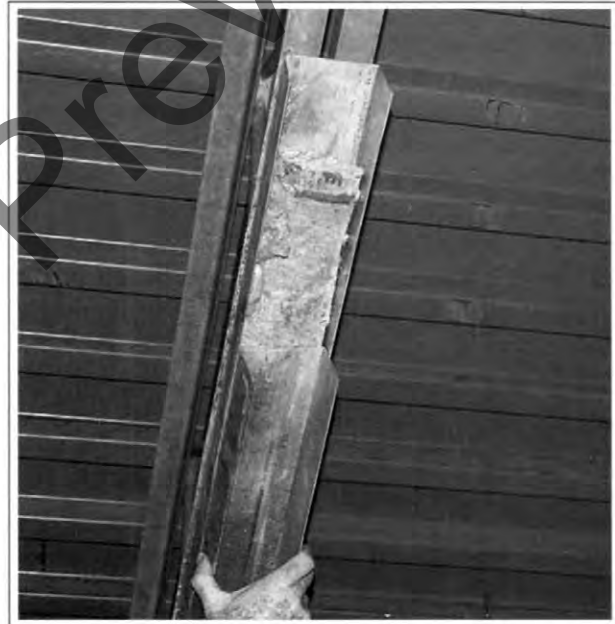
Figure 1-77. The 3\frac{5}{8} -inch-deep leg plate fastened to the bar joist has the safining installed. The second stick of the deflection plate is being installed to hold the dense, heavy insulation in place.
