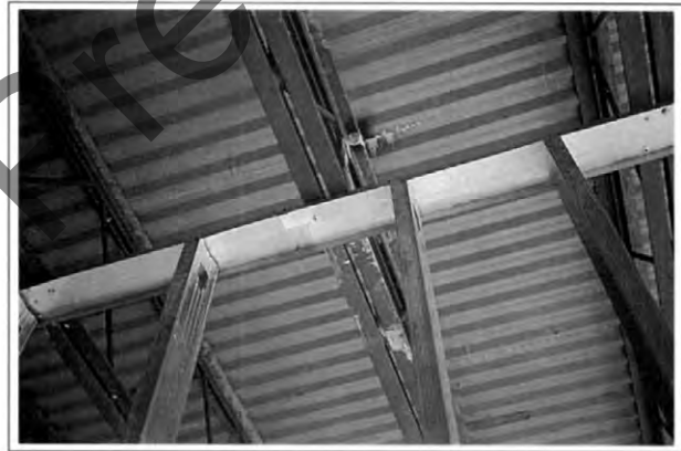
Figure 1-44. The top plate of a 3 5 / 8 -inch wall screwed to the bottom of the bar joist using S-12s (self-drilling framing screws).
