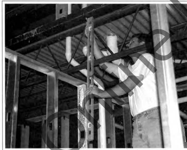
Figure 1-47. Using a 4-foot magnetic level to continue the wall line on up to the deck. If you look closely you can see the bottom of a stud up on the floor above.
