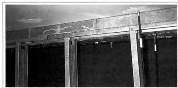
Figure 1-78. Here the deflection plate is formed using deep leg plate for both sections of top plate. The layout studs are screwed off to only the lower section of top plate.
