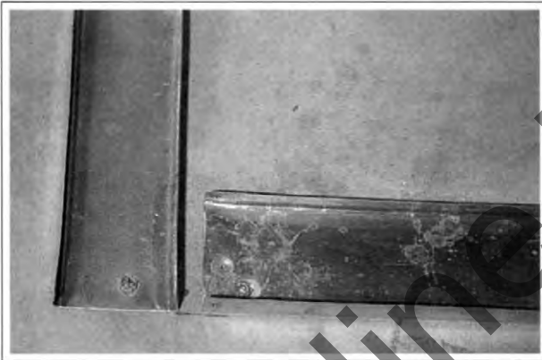
Figure 1-38. Here we see the bottom plate of a 3\frac{5}{8} -inch wall forming an inside/outside corner, leaving a \frac{3}{4} -inch gap for the drywall to slide inside the wall.
