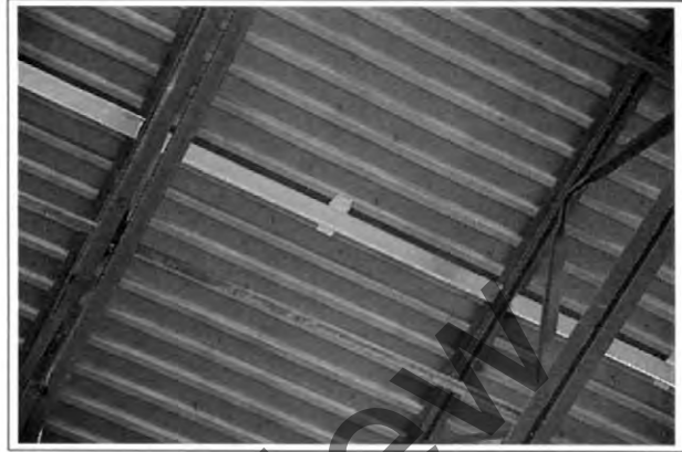
Figure 1-43. The concave grooves in a corrugated metal deck spanned with tabbed plate. The top plate of a 3 5 / 8 -inch wall is screwed in place to the spreaders.
