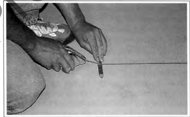
Figure 1-15. Wrapping the chalk line around your pencil not only keeps the chalk line off the floor as it's set to the crow's-foot, it will also keep the line straight over humps in the slab.
