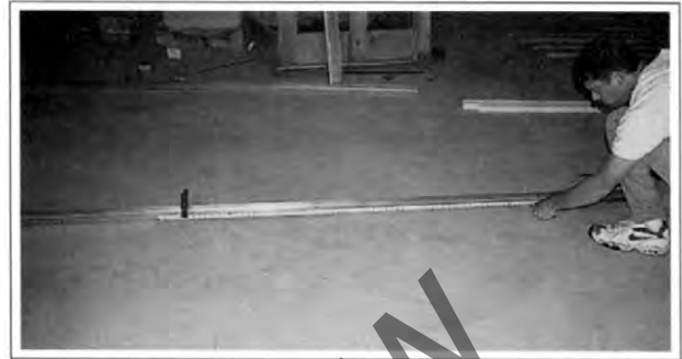
Figure 1-58. This picture shows the end of a tape measure set to a layout mark and clamped to the bottom plate while pulling stud layout.
