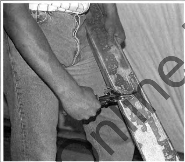
Figure 1-68. Cutting into the hard side of the stud, beginning at the bottom notch mark.
