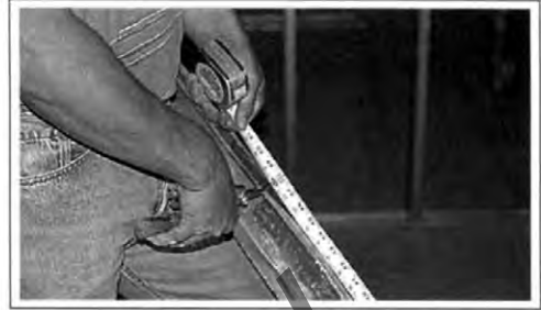
Figure 1-21. Marking the length of the cut with snips.
