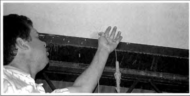
Figure 1-17. The string line of a plumb bob properly run through the fingers and held to the deck with the thumb. Notice that both the wall line plumb point and a 90-degree plumb mark were marked.
