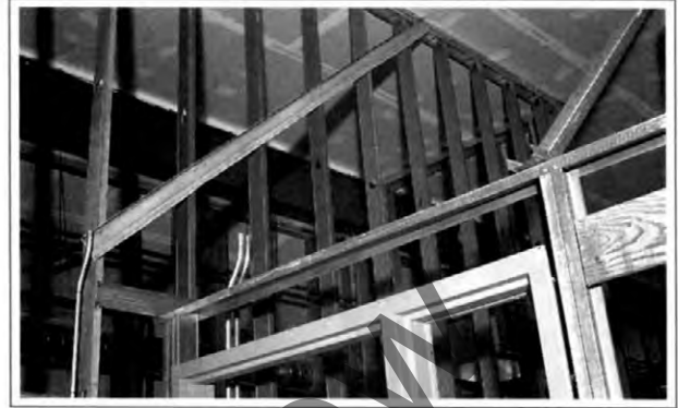
Figure 1-53. A diagonal brace run from the top plate of a tall wall to just above the spreader and top plate of a shorter intersecting wall. The spreader will be taken off as the tall wall is rocked and the slider is tied in.
