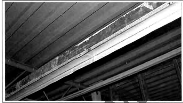
Figure 1-76. This wall is framed to the bar joist using deep leg and standard plate to form a deflection condition. Both sections are spliced, and the lower section is laid out to receive studs.
