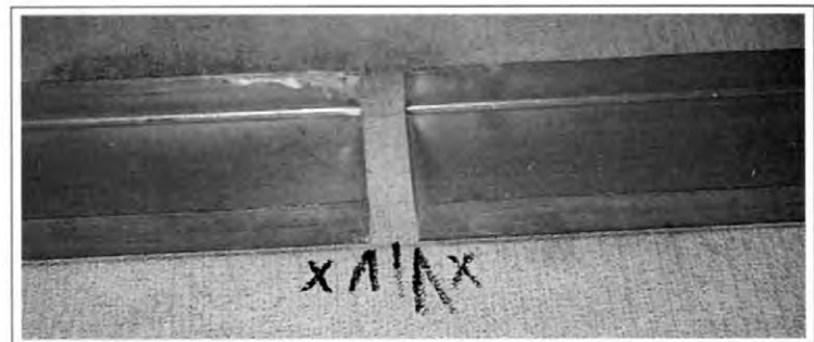
Figure 1-92. Here's the center of the expansion established at the bottom plate, with the plate stopped \frac{3}{8} inch short of the expansion center. The studs will be set hard side to hard side, with the studs right at the ends of the plate.
