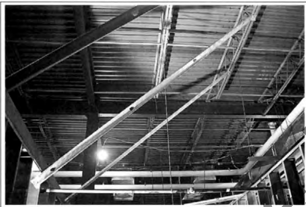
Figure 1-87. Here's a 3 5 / 8 -inch stud used as a kicker. The stud has been twisted before it was clamped to the wall stud to make it stiffer. In contrast, the kicker next to it hasn't been twisted. Both are shot to the bottom of the bar joist.
