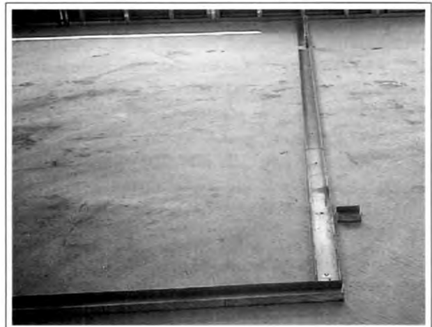
Figure 1-36. The bottom plate of a 3\frac{5}{8} -inch wall stopped for both a corner and a door.
