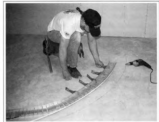
Figure 1-81. In this picture, my partner Kelly is clamping the radius plate to the drywall pattern before screwing it off. The pattern will hold the plate in the form of the radius as it's fastened in place to form the top or bottom plate of a drop.
