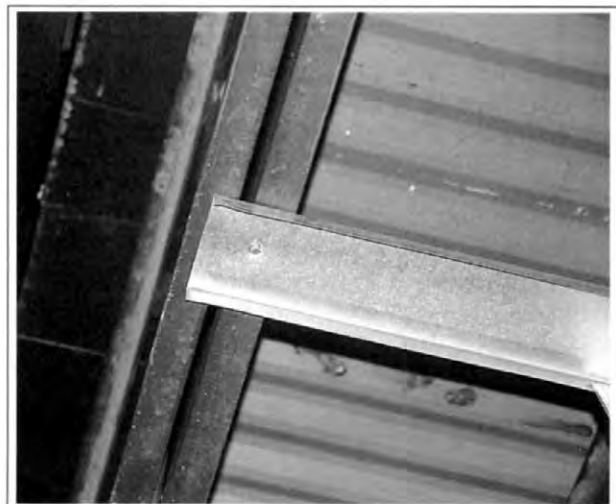
Figure 1-45. Here we see a pin shot right at the bend point of the angle iron at the bottom of the bar joist.
