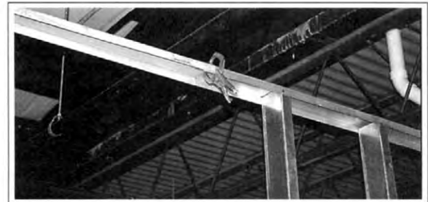
Figure 1-30. A joint in the plate is clamped directly in the corners of the plate.
