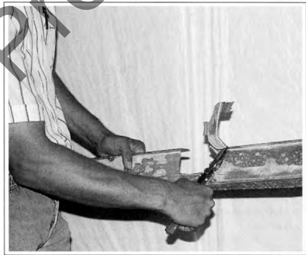
Figure 1-70. The second turn made cutting back out to the edge of the stud to complete the notch.
