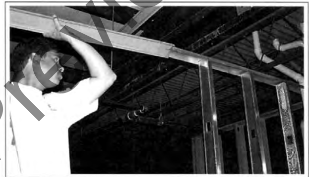
Figure 1-29. The splice will hold up one end of the top plate in this freestanding wall.
