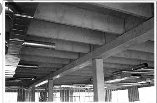
Figure 1-41. This prestressed concrete truss system supports the floor above.
