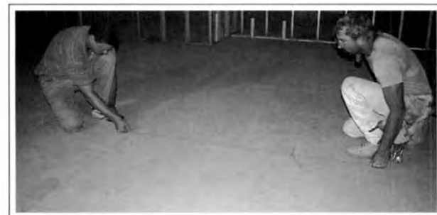
Figure 1-8. Pulling the chalk line from the 3-foot mark through the intersecting arcs completes the 3-4-5 squaring method.
