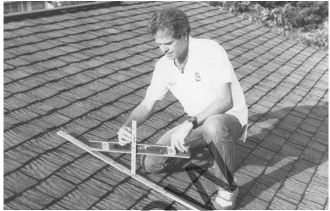
Figure 1-15 Determining roof slope
