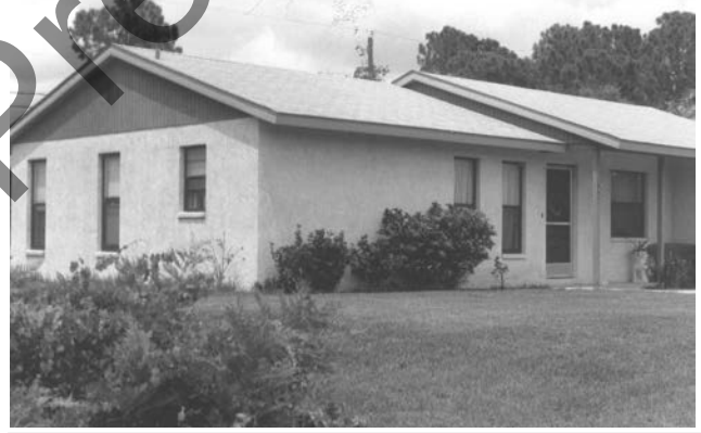
Figure 1-26 Multi-level roof overhang
