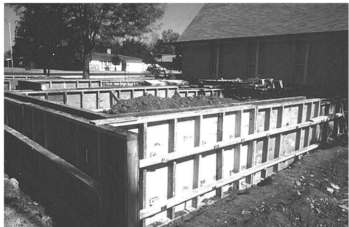
Figure 1-4 Poured concrete wall forms
