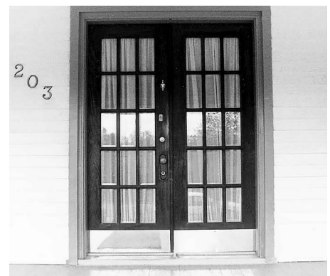
Figure 9-1 Repaired French doors
